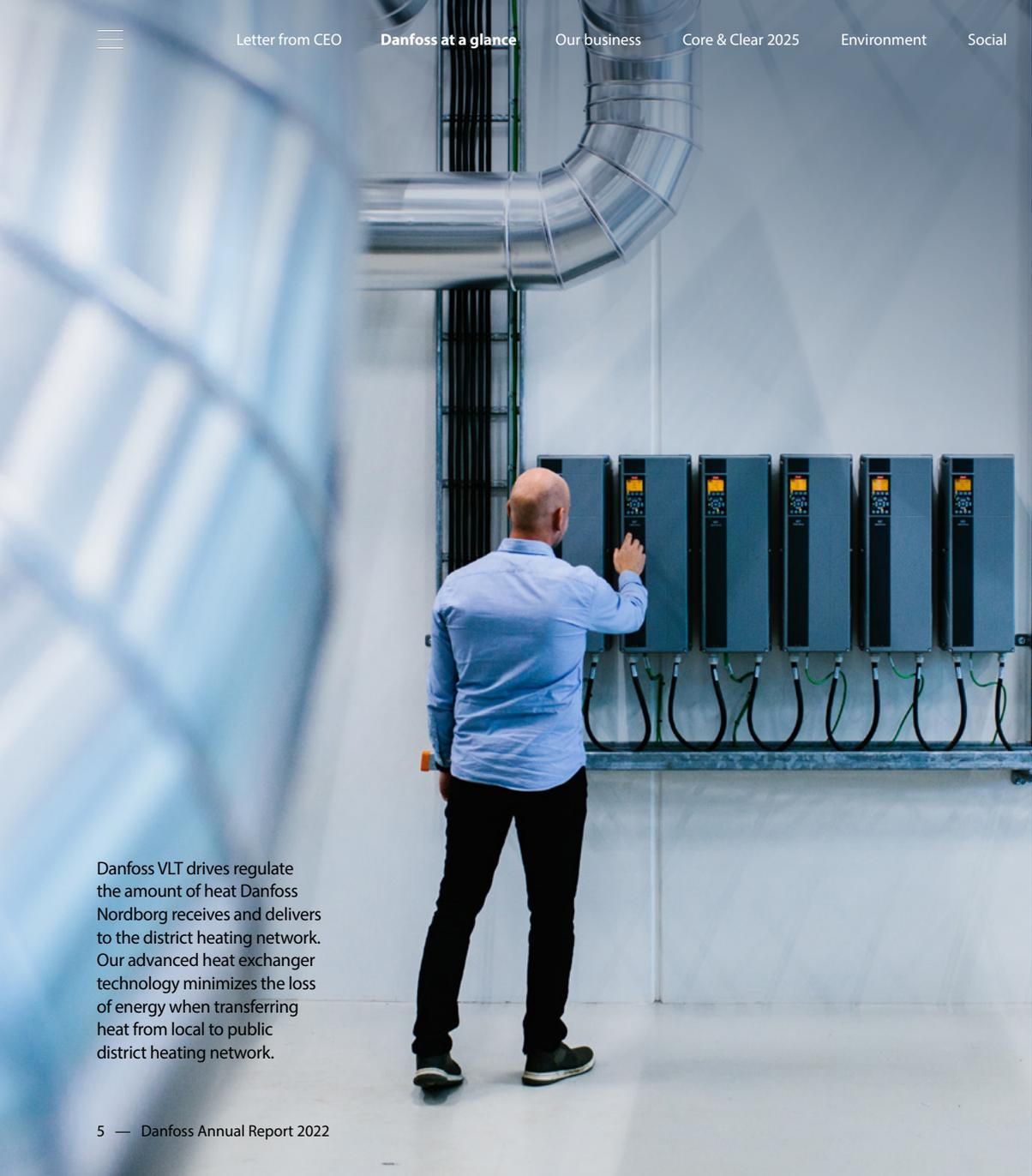
Danfoss VLT drives regulate the amount of heat Danfoss Nordborg receives and delivers to the district heating network. Our advanced heat exchanger technology minimizes the loss of energy when transferring heat from local to public district heating network.
